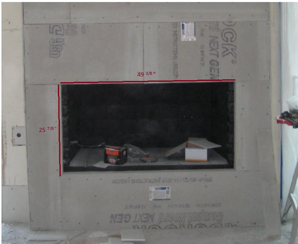
3. The end goal is to have a fire place that has tiles on the entire face, and an **aluminum** firebox frame with the following dimensions:
